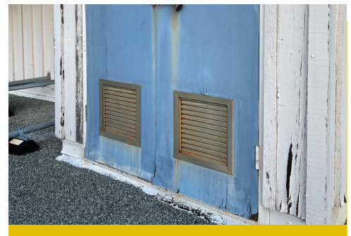
Weathered and damaged doors at West Elementary School.
